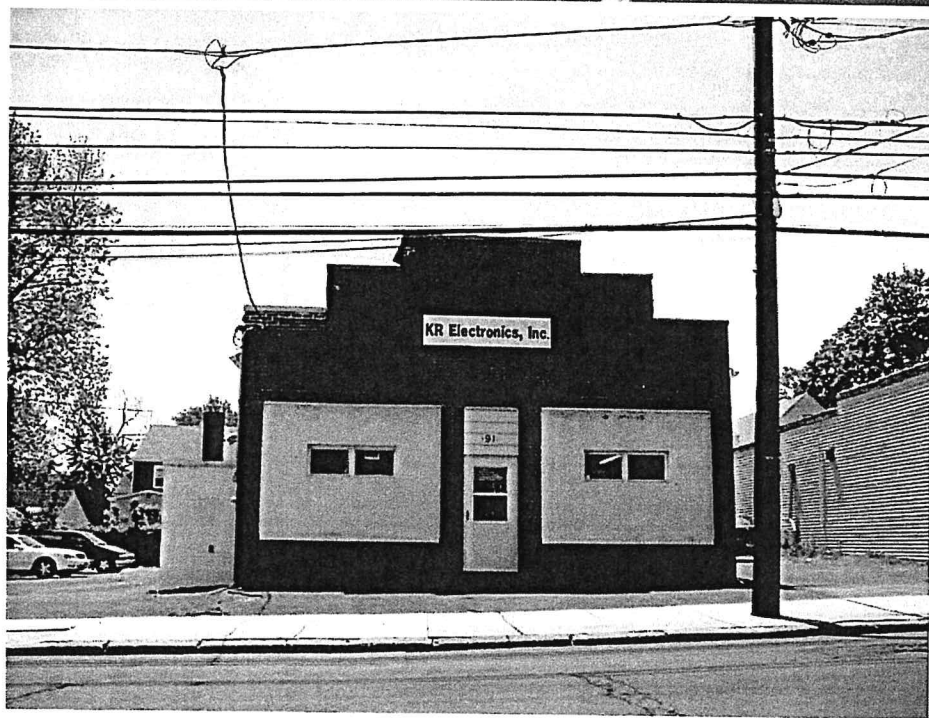
Typical facade - older commercial property
