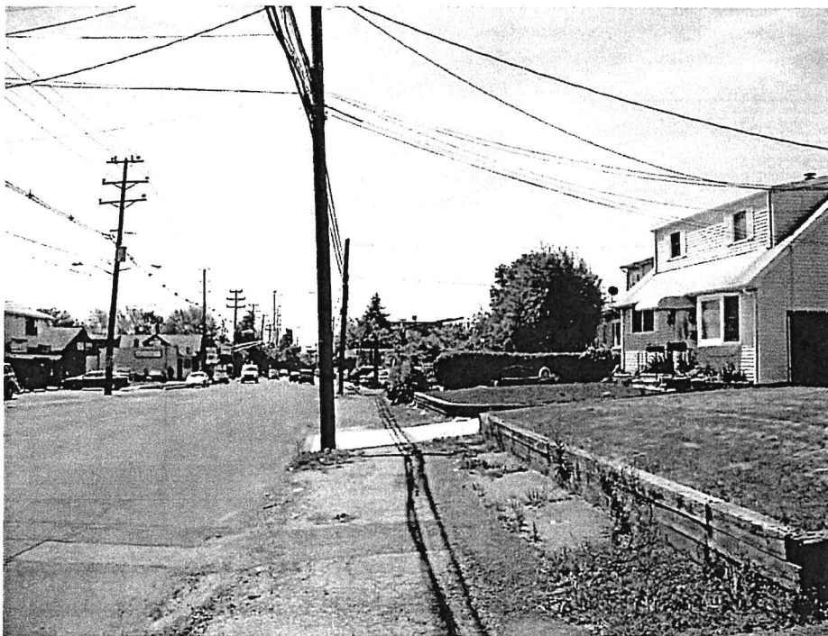
Need for sidewalk improvements
