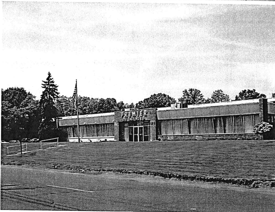
Light-industrial / manufacturing use across from single family residences
